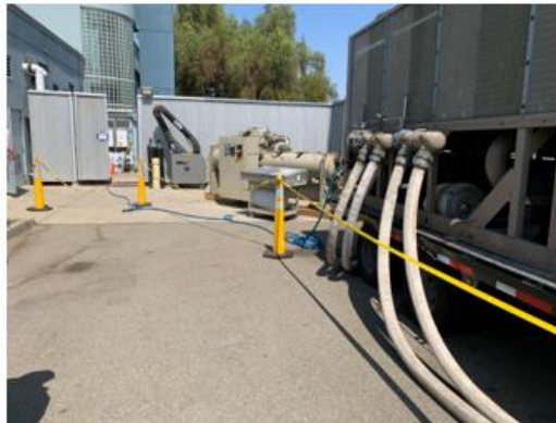
Temporary Chiller startup
