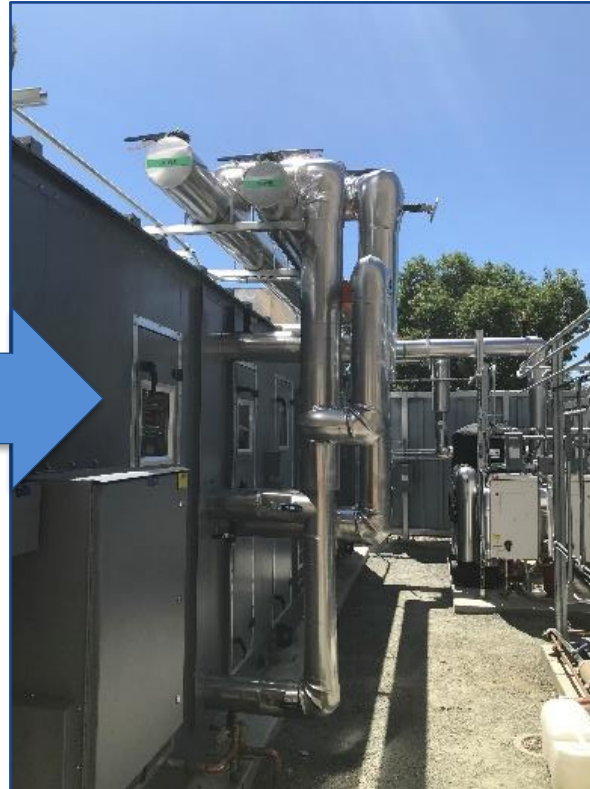
New ACU-08 installed at ground level
