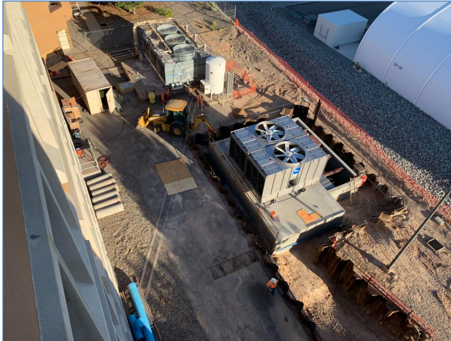
Construction in progress; existing unit on left, new replacement on right.
